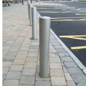
Stainless Steel Bollards- Fixed (c/w Base Plates) 1mHX101mmDia- Unit Cost = c. €295.00 each
